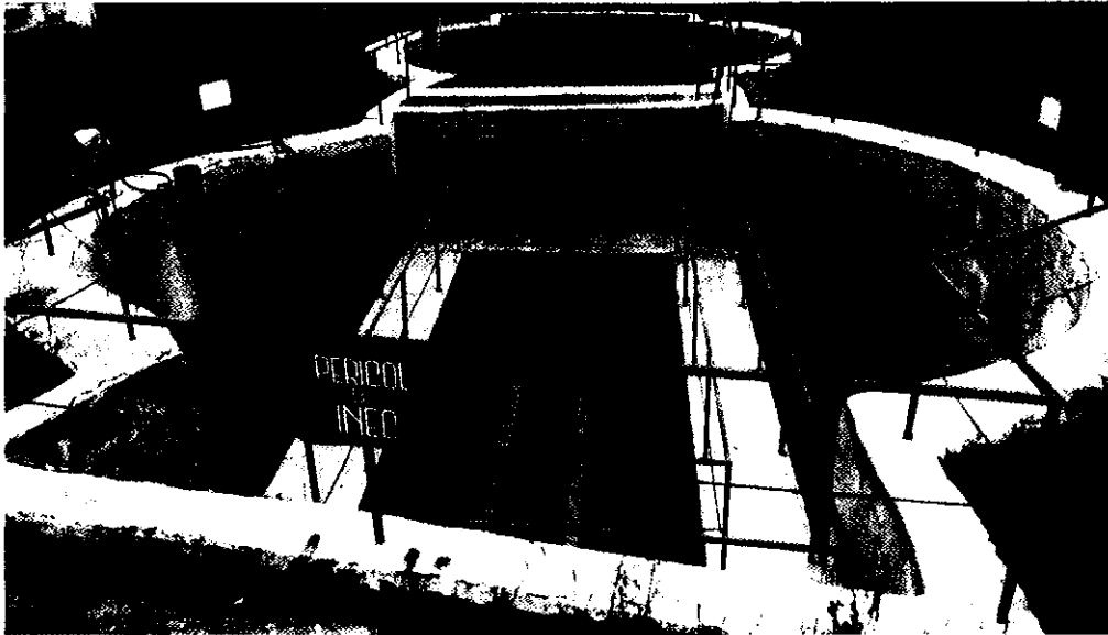
Figure 5-125: WWTP Targu Ocna
