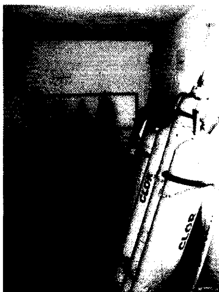
Figure 5-87: Storage for chlorine gas at RSV 1,000 m 3
